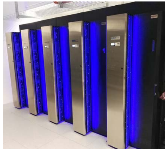
Backside: Cooled backdoors
