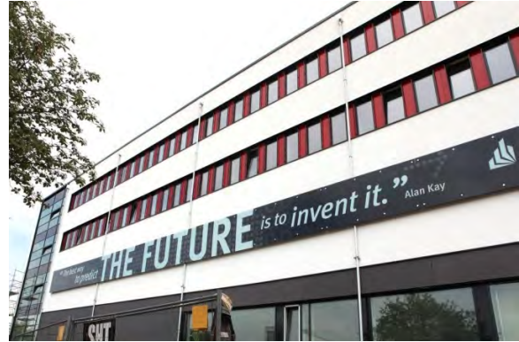
Fig. 2: Building O. The compute center is located behind the Alan Kay quote
