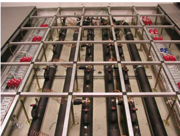
Fig. 7: Tichelmann ring and power supply of OCuLUS
